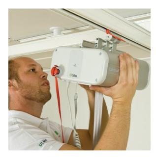
Moving the Lift Motor (excluding LR242 S and LR 242 ES) The Quick-Release Hook™ Carriage makes it easy to move the system between rooms.
